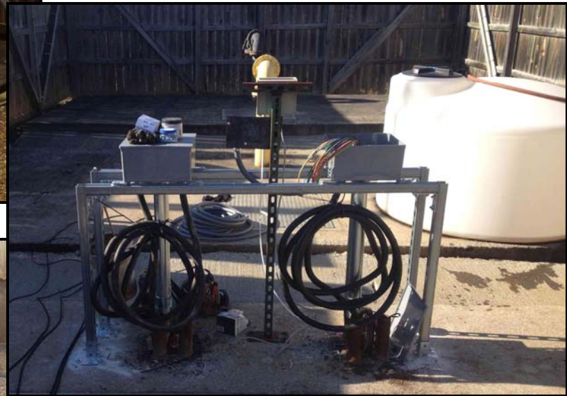
Photo 5 – Existing Midway Wastewater Pump Station Chemical Tank & Surge Tank Tops
