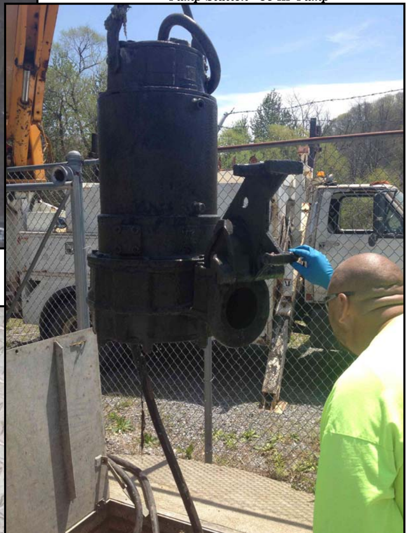
Photo 8 – Brush Fork Wastewater Pump Station - 60 HP Pump
