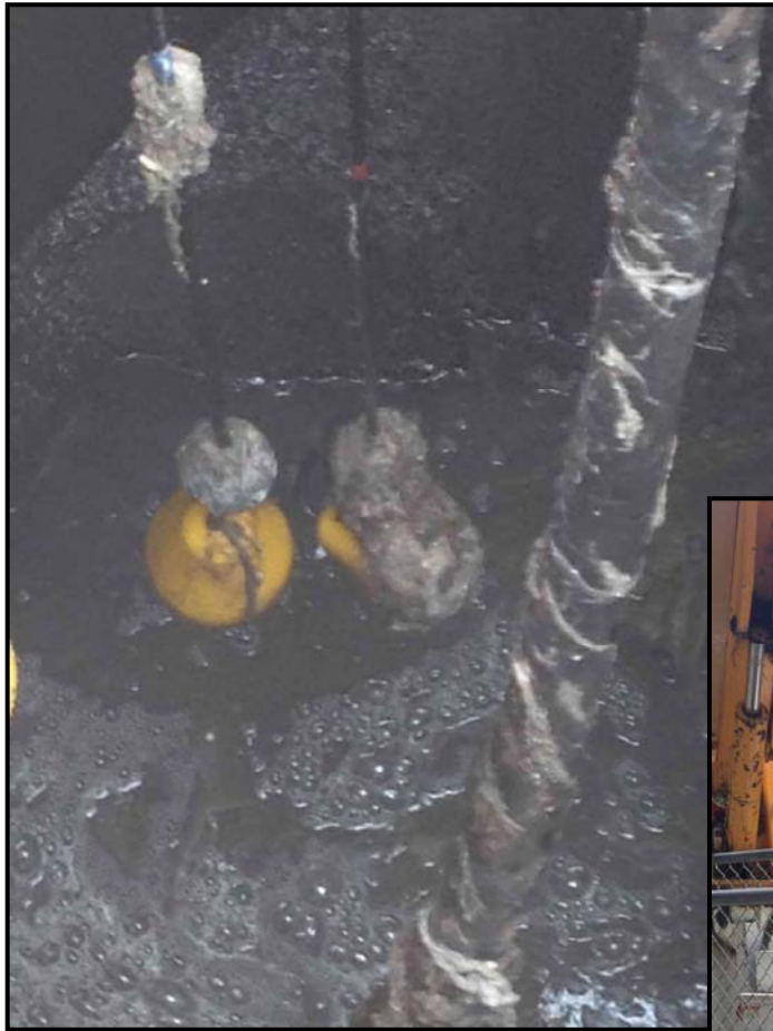
Photo 7 – Brush Fork Wastewater Pump Station Hung Float
