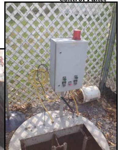
Photo 10 – Copolla Wastewater Pump Station Control Panel
