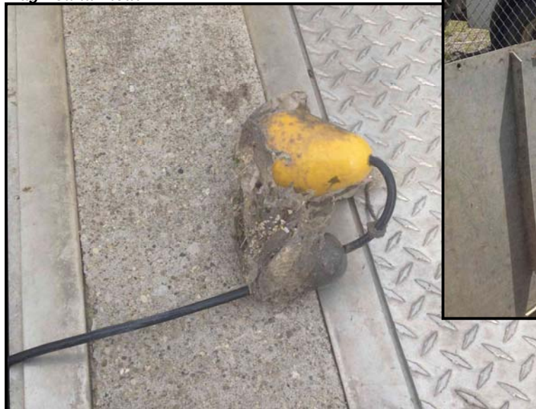
Photo 9 – Brush Fork Wastewater Pump Station Rag Bound Float
